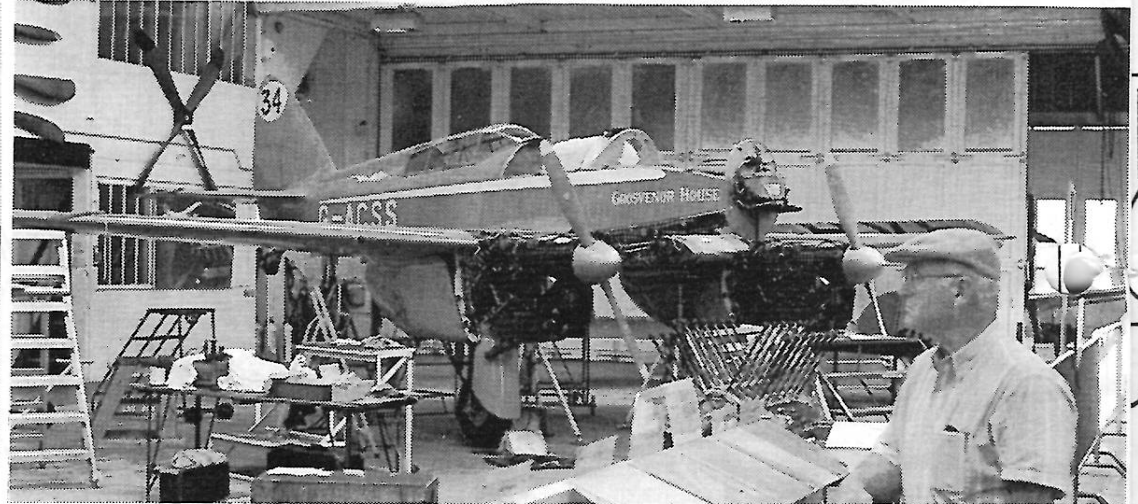
Hurst Bowers reviewing the rebuilding of the Grovesnor House at Old Warden.
