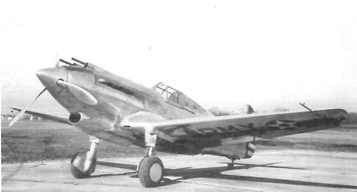
THE XP-40 WITH INTERMEDIATE RADIATOR INSTALLATION.
